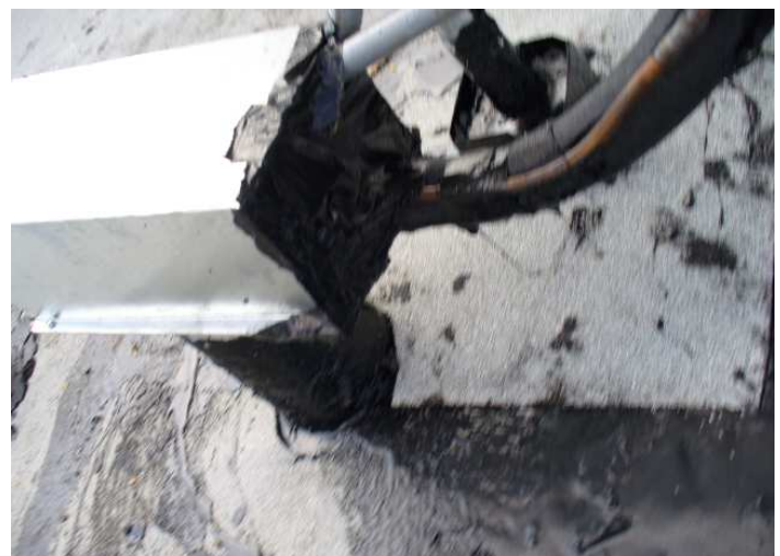
The chase for the condensing unit.
