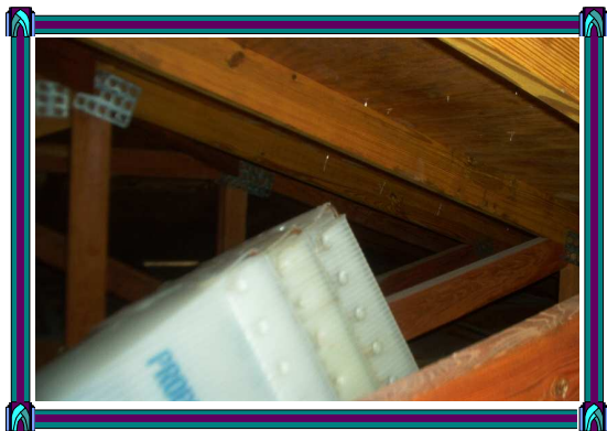
The remaining pictures are of the missed nails mentioned on the roof inspection report.
