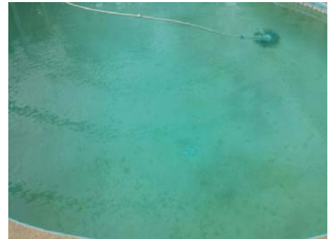
Pool surface was pitted in several areas and requires re-coating.
