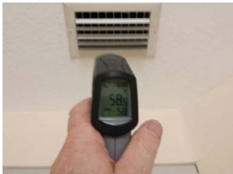
Cooling cycle being tested.
