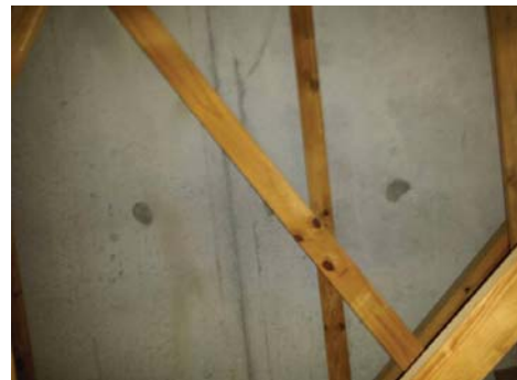
Concrete walls (poured in place) in attic.
