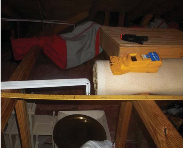
Truss spacing
