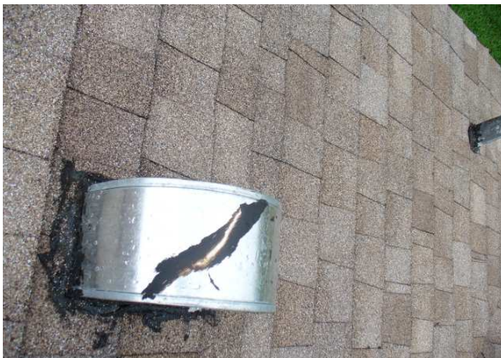
Cold process roof cement on vent.
