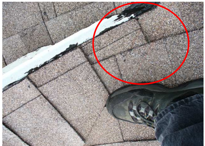
Cold process roof cement at valley.
