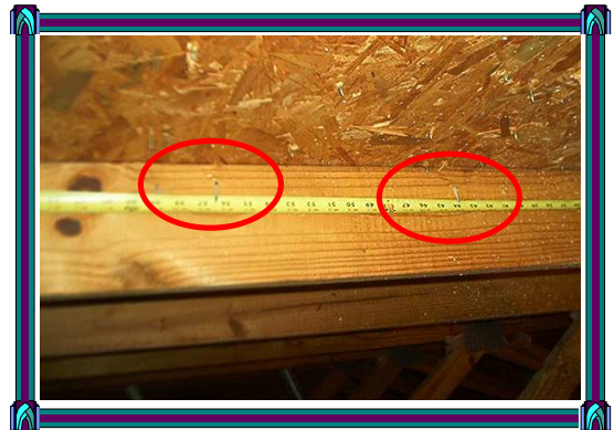
This does not conform to the local building code pertaining to the nailing pattern.
