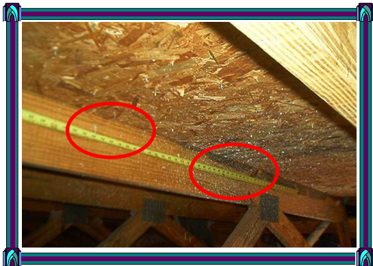
The following three pages of pictures show the numerous missed studs in the attic.
