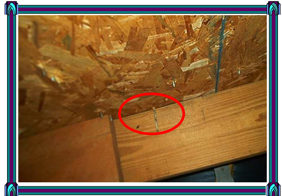
This does not conform to the local building code pertaining to the nailing pattern.
