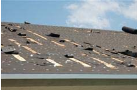
Roof nail repairs.
