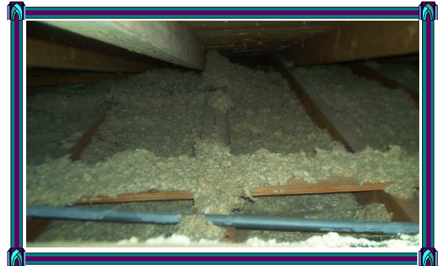
Wood rot at decking at front valley.
