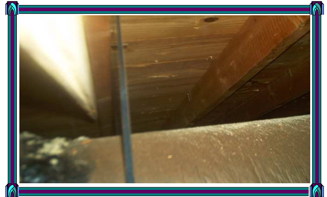
Other beam that is not secured to support wall.
